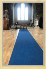
the recent replacement of the old floor. The floor boards had deteriorated to a serious extent, posing a safety issue to our parishioners and visitors. The new floor is constructed with warm oak timber boards with a carpet centre aisle. It was engineered with a concrete base which was
