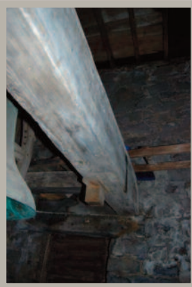
One of the two pitch pine supporting beams
