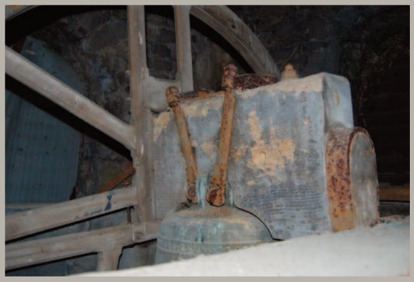
View of decayed headstock
