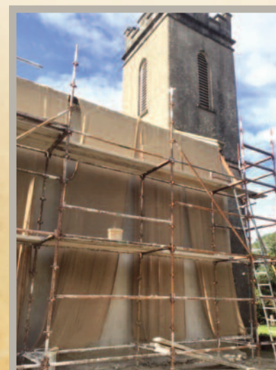
The lime rendering of the walls at St. Thomas's Church Moyard
